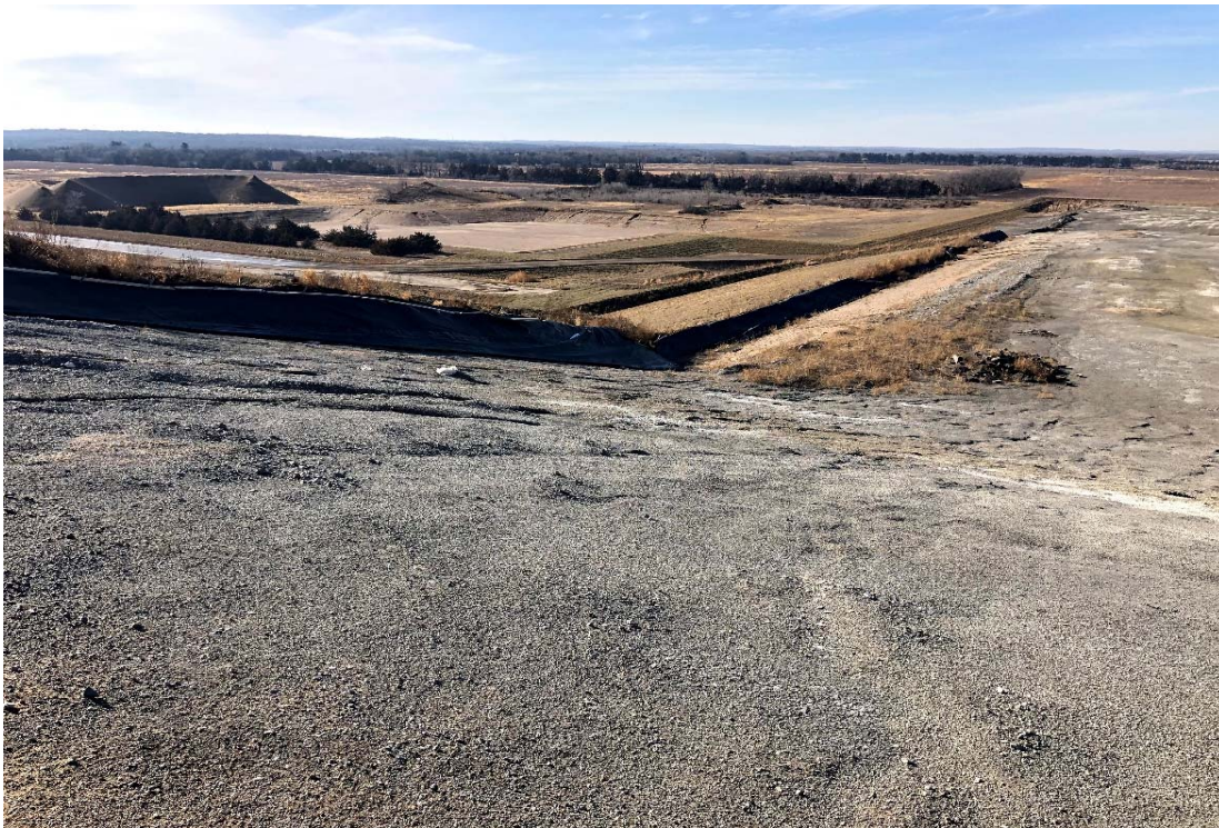
Photo 2 Run-on/run-off containment berm in foreground, looking southwest. Future cell excavation area in background. 11/19/2020
