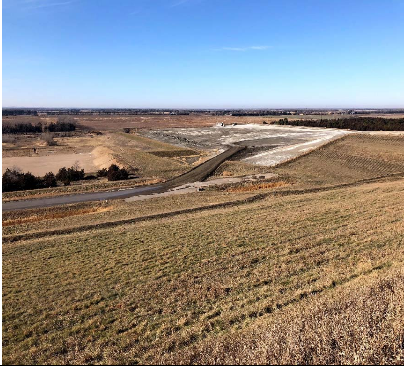
Photo 1 Left: excavation of future landfill cell. Right: existing final cover and active cell, looking northwest. 11/19/2020
